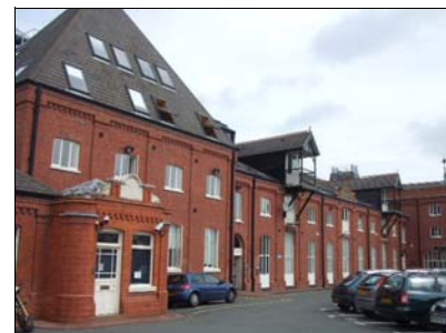
Prospect House, Belle Vue Road, Shrewsbury
