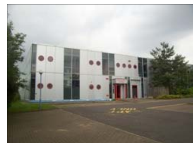
Kingsland House, Stafford Court, Telford
